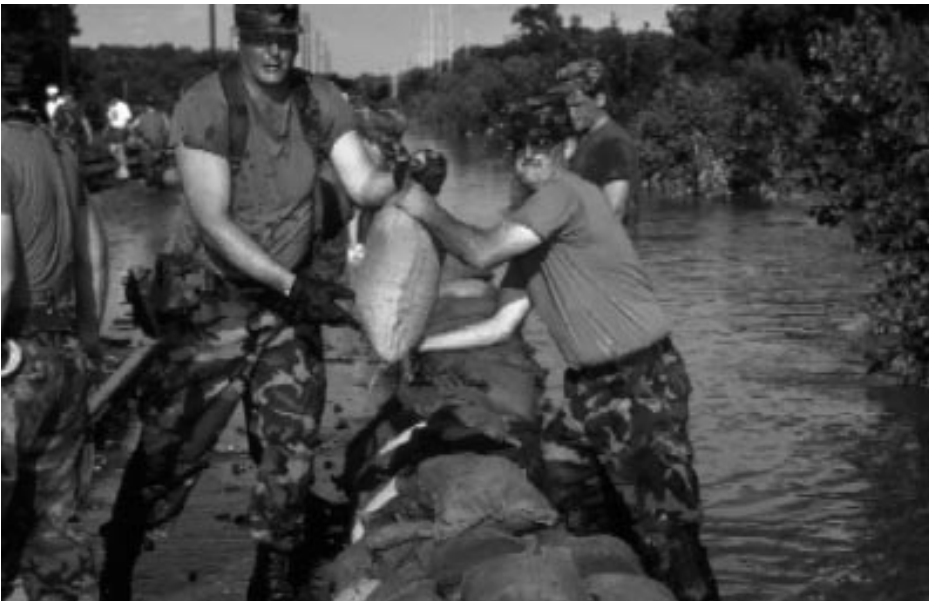
Civilian volunteers and National Guard personnel build a sandbag levee at Valley Junction, Iowa, trying to stop flooding of the Raccoon River in July 1993.
